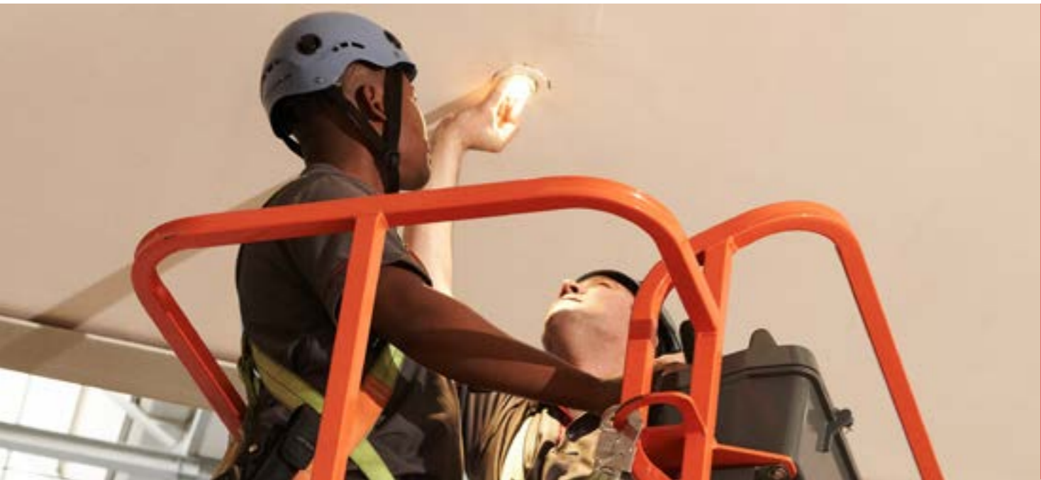
Retrofitting ensures sustainable energy efficiency
